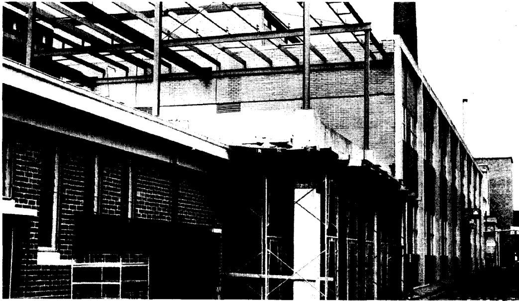
Biology Research Unit Extensions in progress.
