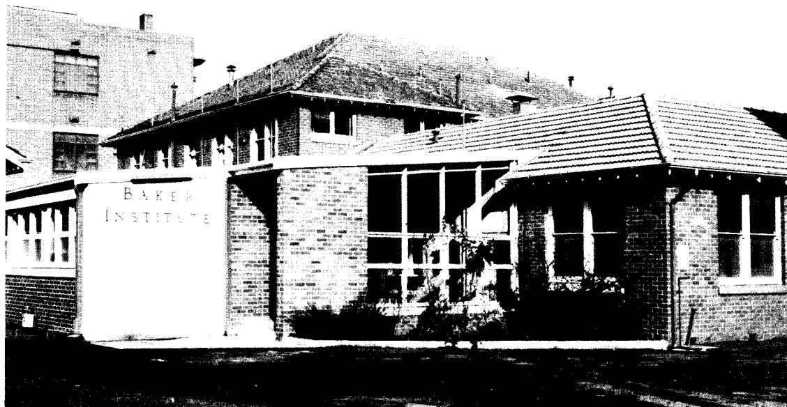
The original building and walkway connecting Institute with Clinical Research Unit.
